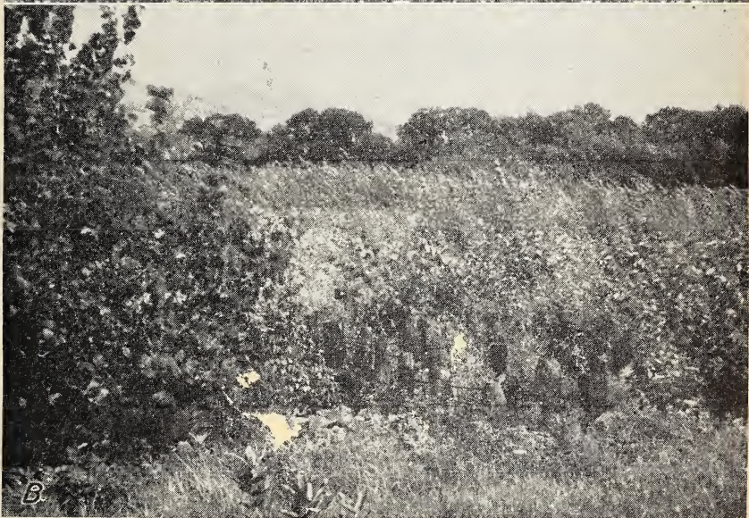
FIGURE 13.—Log-pile check dam constructed in new channel just below main barricade: A , Just after construction in 1938 showing stone apron; B , 4 years later showing growth of buffer planting.
